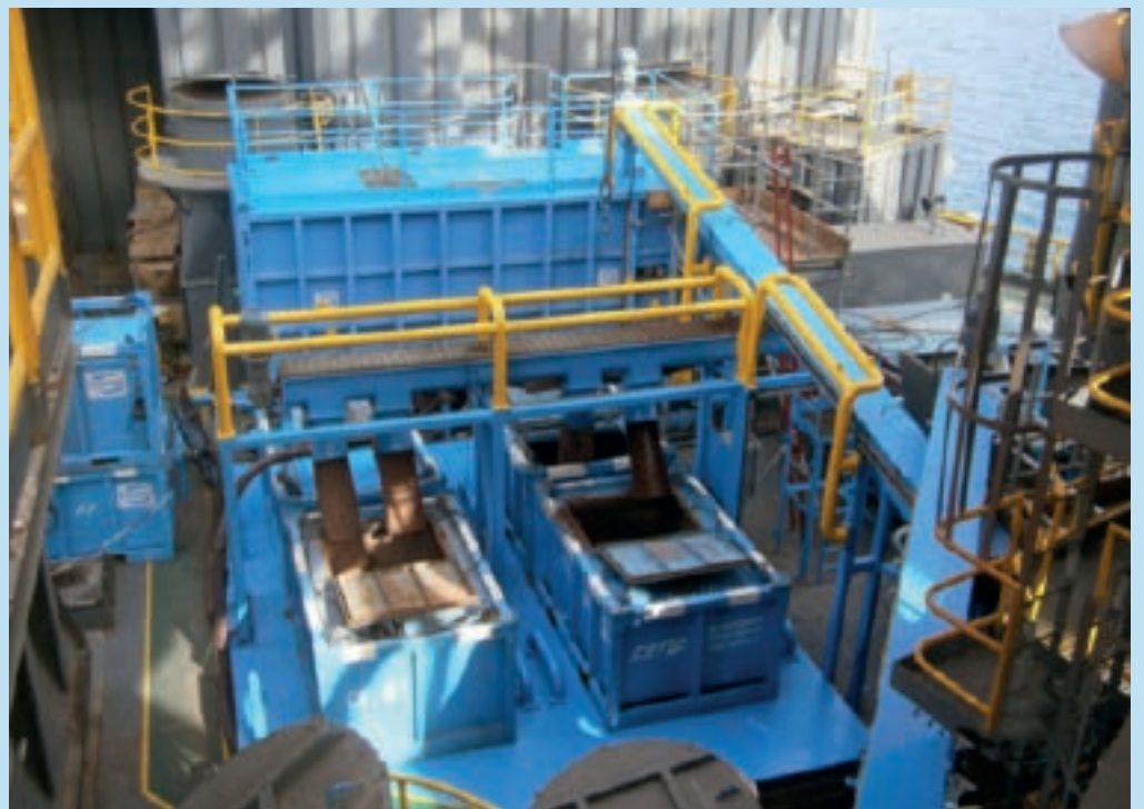
TWMA skip-filling station and CCDS installed offshore
