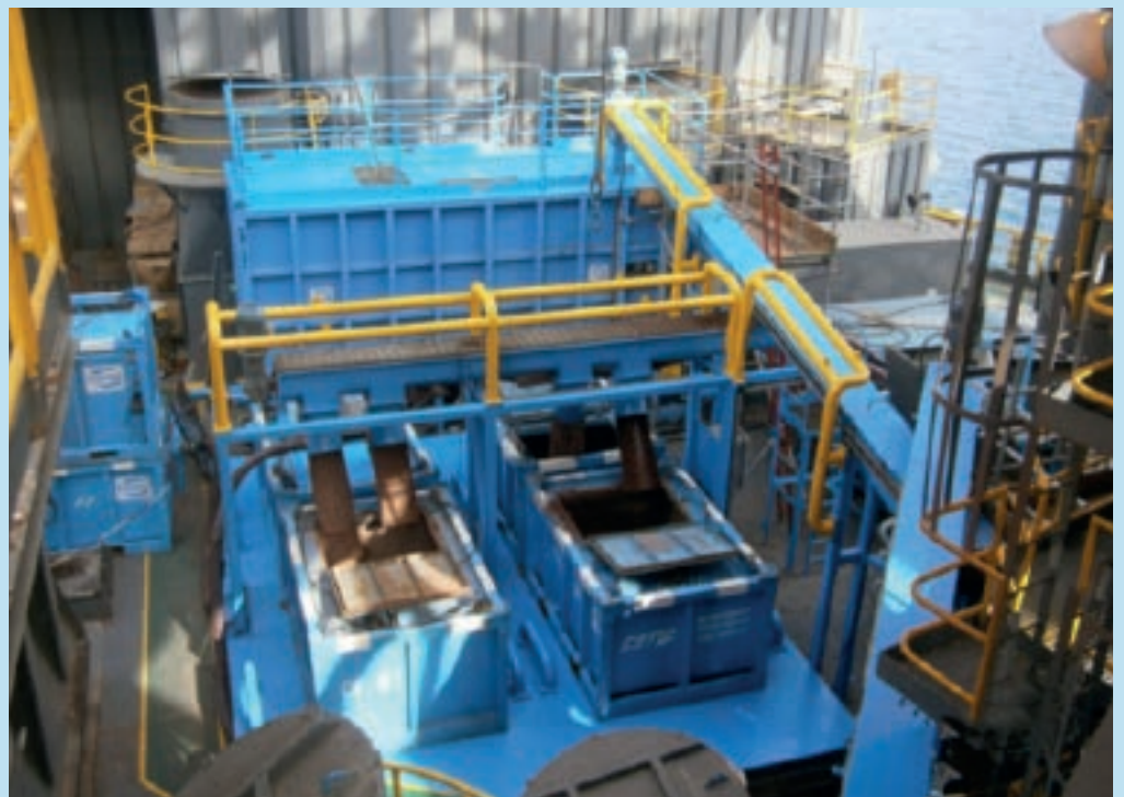
TWMA skip-filling station and CCDS installed offshore
