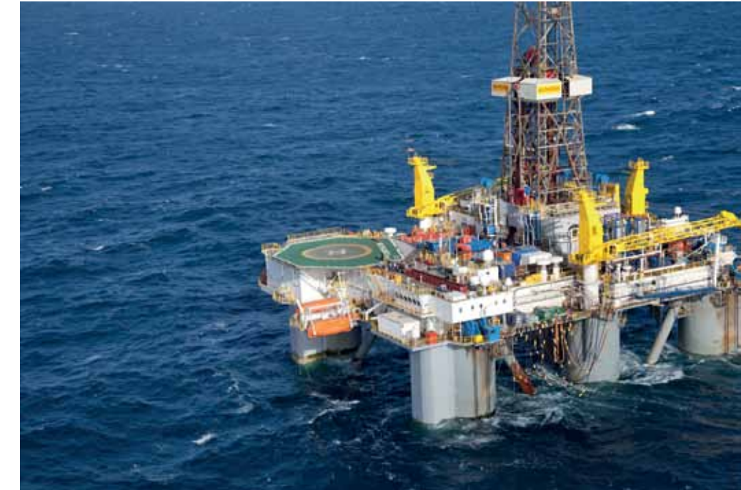
The WilPhoenix semi-submersible rig
